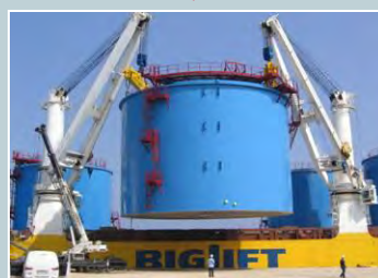
Tanko Italia MEG-Tanks: 1 300 tons
