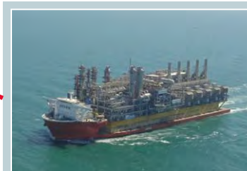
Dragados Process plant 35 000 tons
