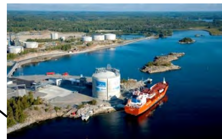
LNG Import Terminal in Nynäshamn operated by AGA
