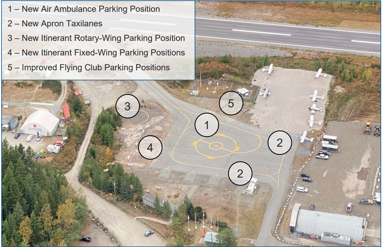
Completed apron management improvements (Photo courtesy of Sea to Sky Air)
