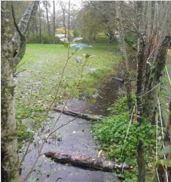
Photo 6: Looking north along west ditch at high water. October 23, 2014.
