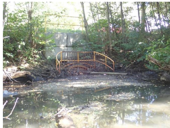
Downstream view of the Mamquam Blind Channel Segment 1, note left bank cattail ( left ); View of modified shallow water community at Buckley Road culvert where persistent debris has partially plugged the culvert ( right ).
