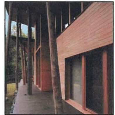
Use of timber in building facades. Form and design should respond to the climatic requirements and reflect the overall theme of the development where appropriate
