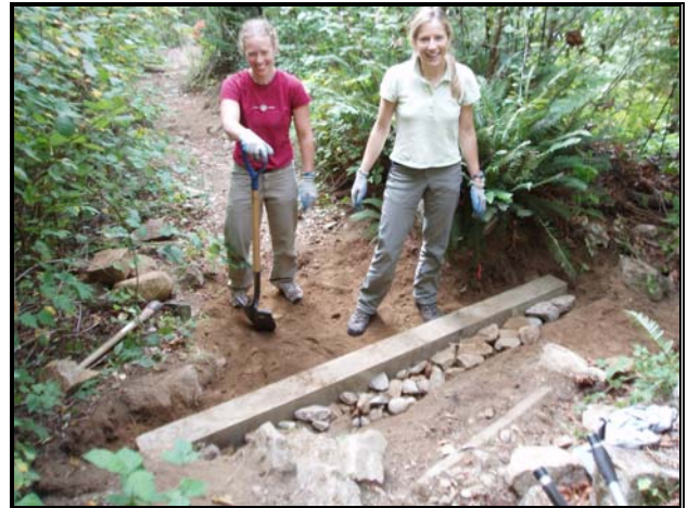
Volunteers making trail drainage improvements, September 2005 “Adopt-a-Crag” event
