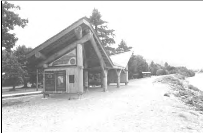
Squamish River dyke at eagle viewing area
