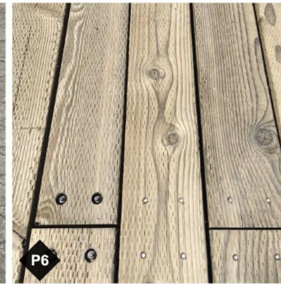
P6 TIMBER DECKING
