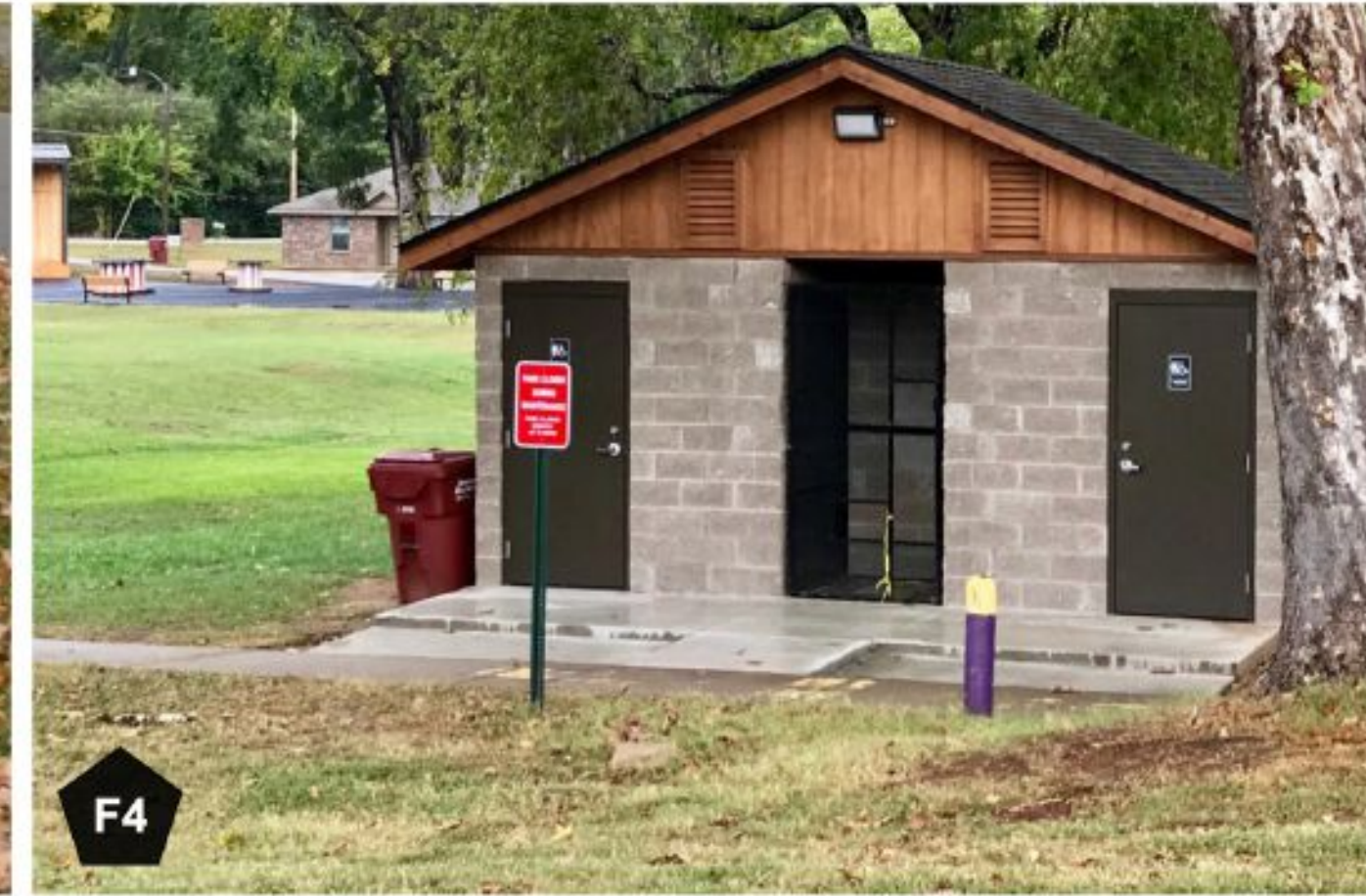
F4 WASHROOM - 2 PAX
