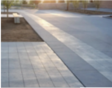
Ex. Concrete banding
