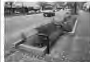
Curbed planting bed in North Vancouver, BC that allows rainwater to infiltrate through curb cuts.
