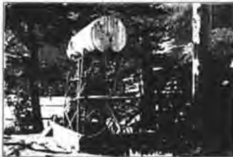
XVIII - DIESEL TANK AND CONTAINMENT BERM Should any hydrocarbon-contaminated soil exist, it will be removed to an approved site.
