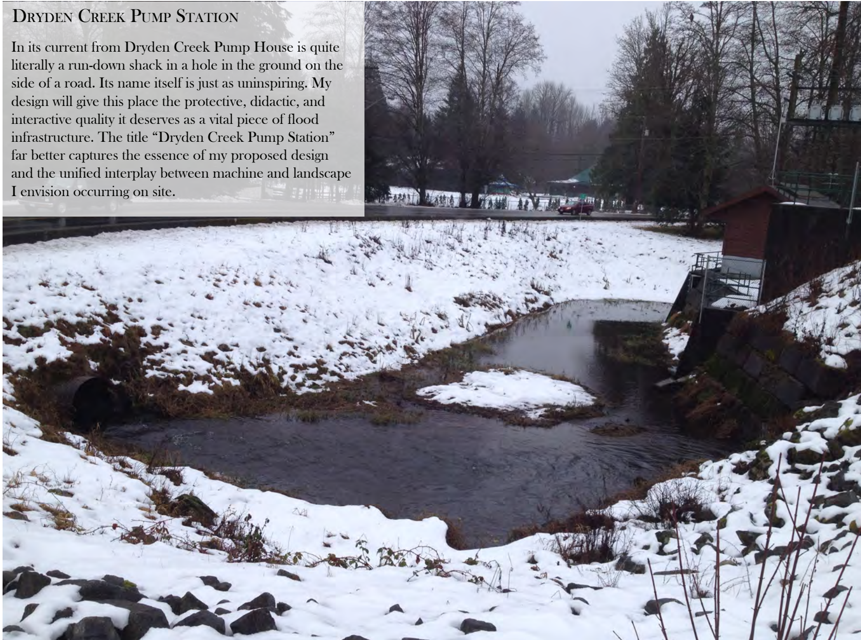
(Figure 6.26) Dryden Creek Pump House: A run-down shack in a hole in the ground on the side of a road.
