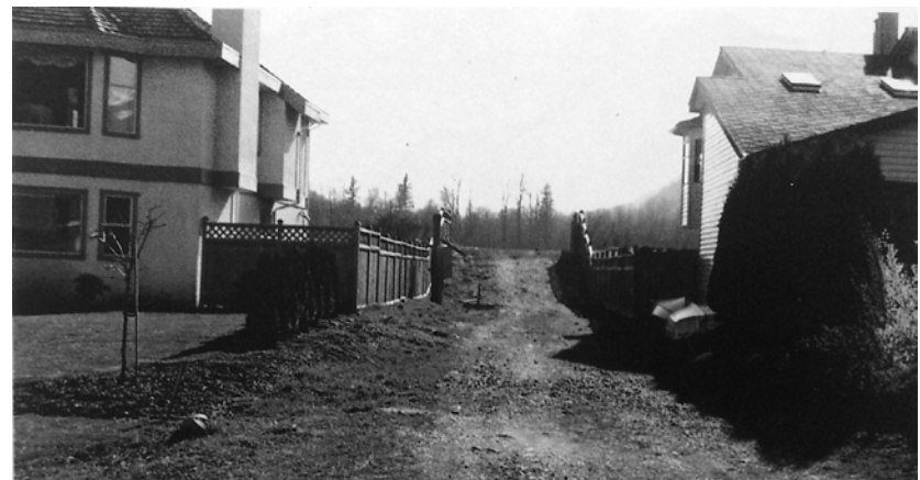
(Figure 5.9): Underground Eagle Run Pump Station Right of Way (Image: Kerr Wood Leidel, 1992: Appendix A)
