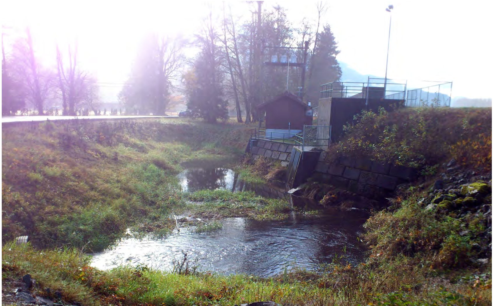
(Figure 5.11): Dryden Creek Pump House with forebay and culvert
