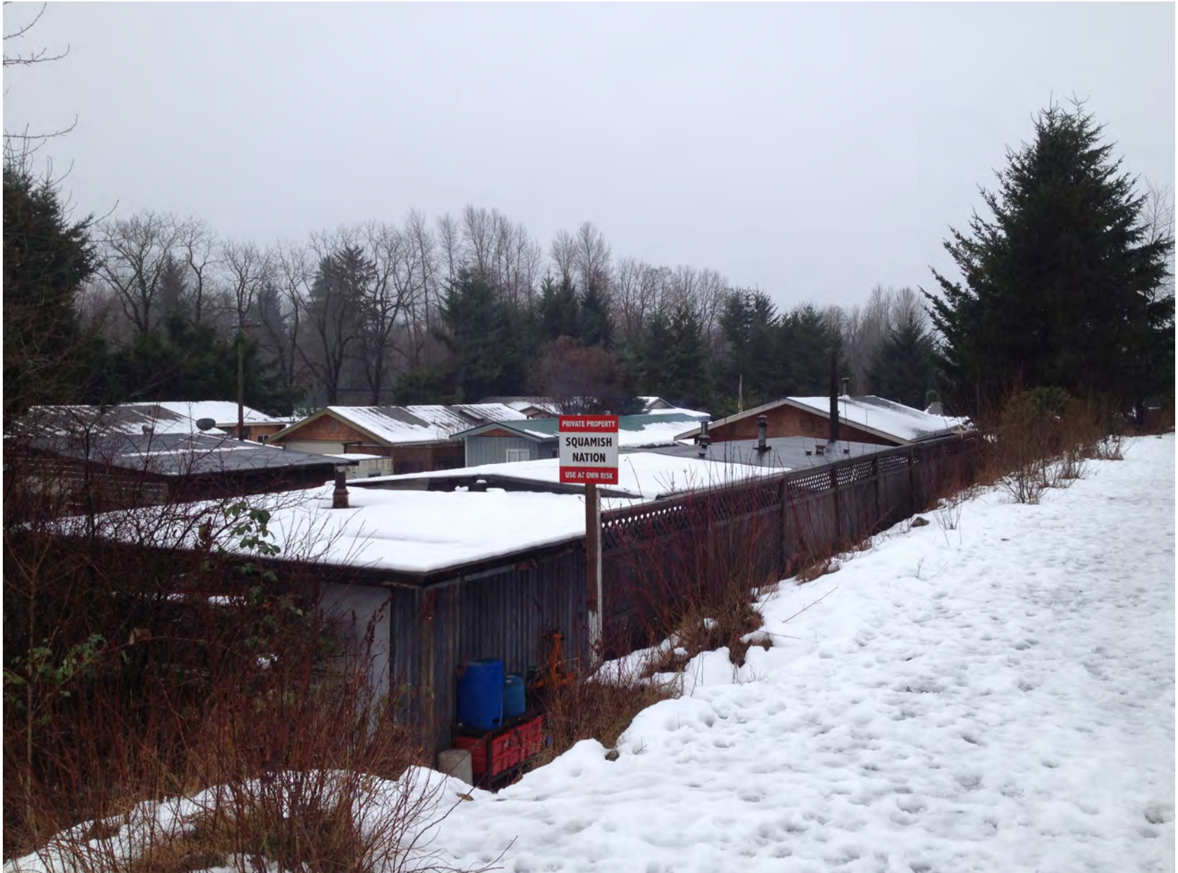
(Figure 6.14): The Squamish Nation community at the foot of the dike is in a position of significant flood vulnerability.
