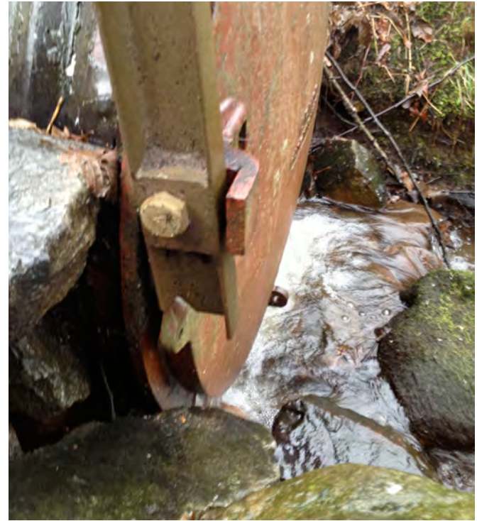
(Figure 6.5): Horse Creek Outlet releasing water to the river
