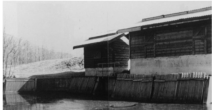
(Figure 5.8): Judd Slough Pump House (Image: Kerr Wood Leidel, 1992: Appendix A)
