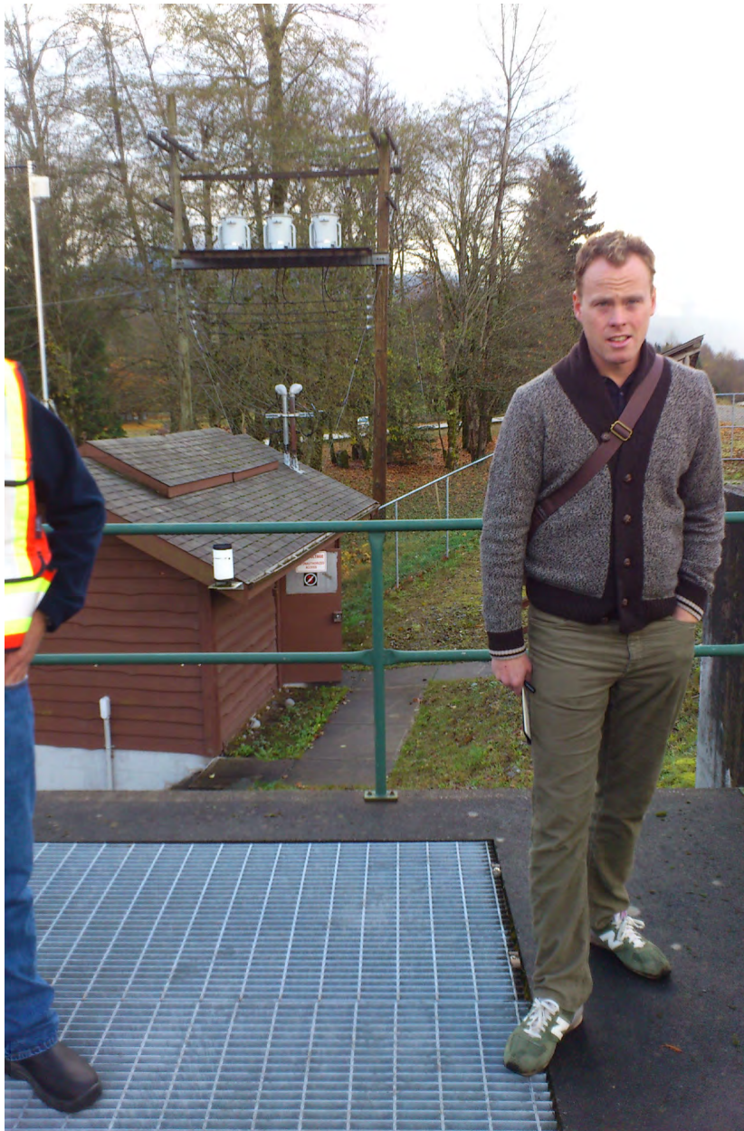
(Figure 5.15): Man standing on top of Flygt VFD Submersible pump housing. There is one unit in this housing with a cavity for the expected second (Kerr Wood Leidel, 2012).
