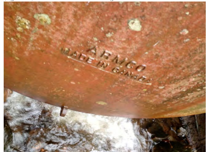
(Figure 6.6): A weathered-steel artifact in the floodplain wilderness.
