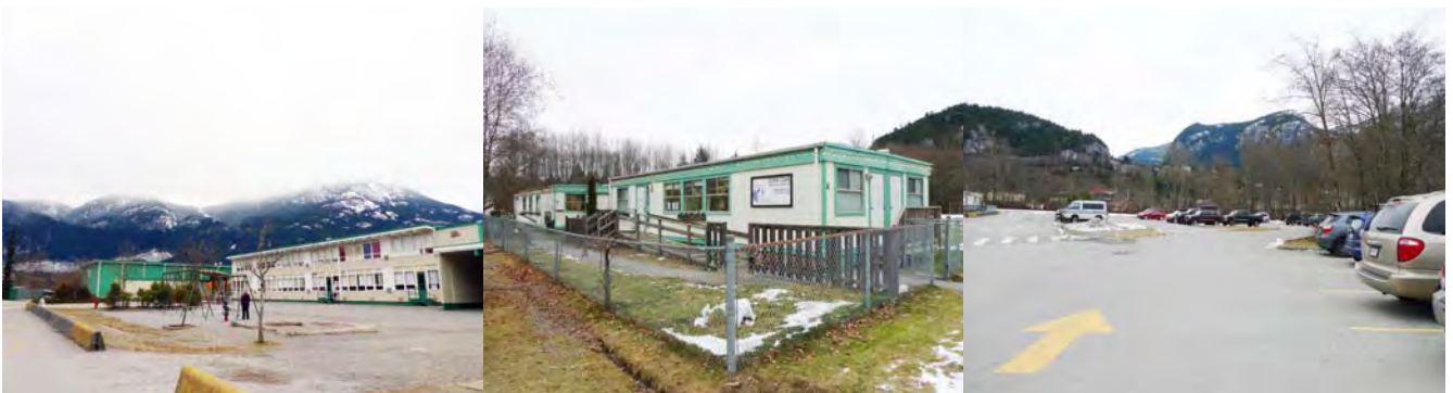
Squamish Elementary School
