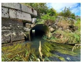
Photo 17 – Dryden Creek – Culvert inlet conveying flow under existing dike.
